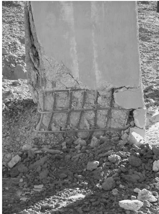
Figure 4.4: Deflection and spall of test column (Williamson et al. 2010)
